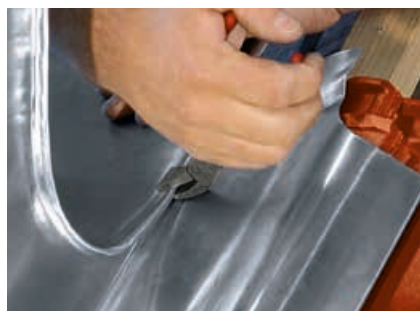
Seam preparation for back apron
