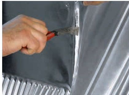
Preparing the single seam
