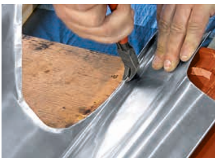
Seam preparation for side flashing
