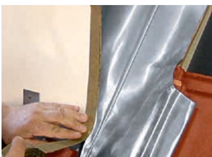
Using an adhesive strip
