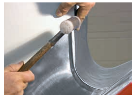
Seam completion
