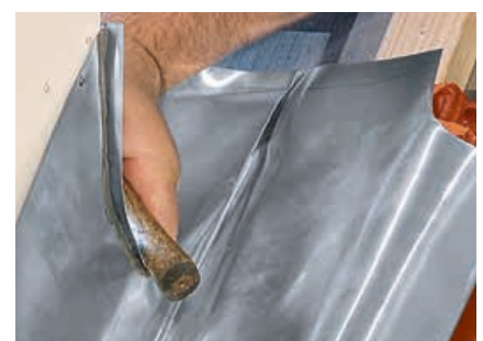
Grouting the back apron/side flashing
