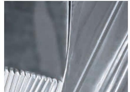
Completing the single seam
