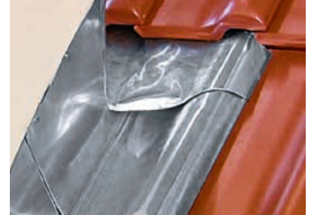
Ridge-side connection, overlapped
